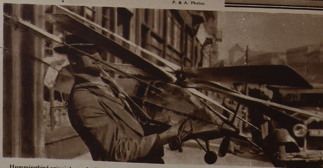
Hummingbird principles embodied in new plane. Valentine Newbauer, of Los Angeles, has built an airplane, the outstanding feature of which is its ability to rise vertically from the ground and to descend in the same manner, with the motors cut off. This is accomplished by a double set of four-bladed revolving wings attached to the top. With the aid of other devices the plane can dart from side to side and move backward and forward.
