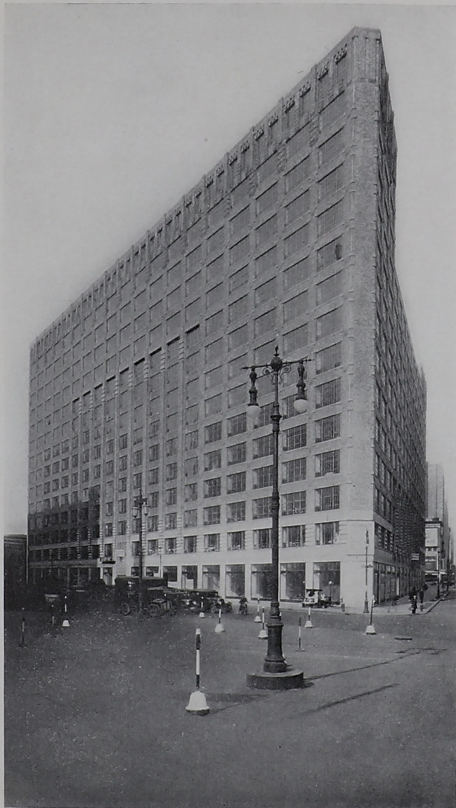
HOLLAND PLAZA BUILDING CANAL, VARICK, WATTS, AND HUDSON STREETS Owner: York Investing Corporation Builders: Schroder and Koppel Architect: Buchman and Kahn
