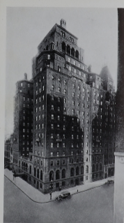
ALLERTON HOUSE MADISON AVENUE AT 38TH STREET Owner and Builder: Altrion 38th Street Corporation Architect: Margatsoy and Ogden
