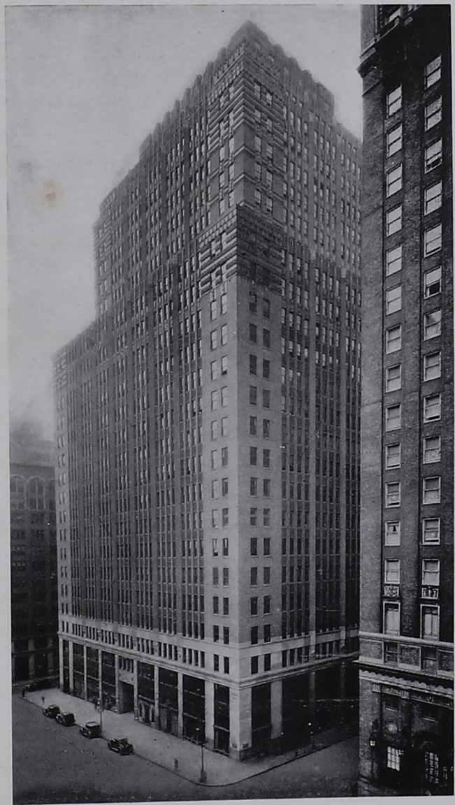
2 PARK AVENUE Owner: 2 Park Avenue Corporation Builders: Schroder and Koppel Architect: Buchman and Kahn
