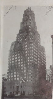
KOEBERICH MUSEUM RIVERSIDE DRIVE AT 103RD STREET Builder: Longacre Engineering and Construction Co. Architects: Sagorwan and Berger Reinke, Corbett and Harrison } Associated
