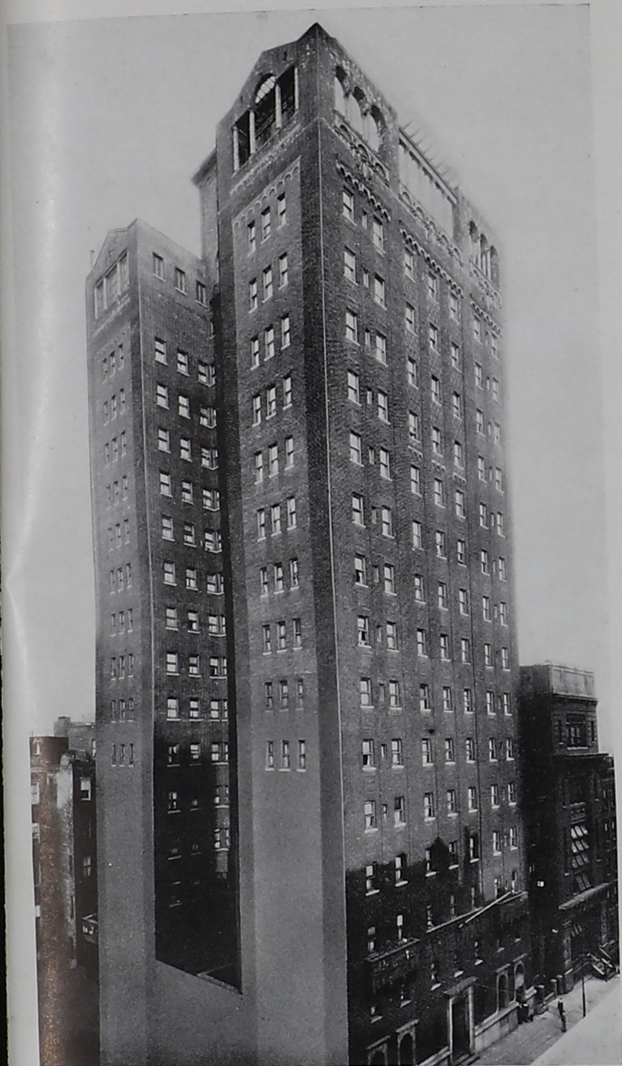
ALLERTON HOUSE 149 EAST 39TH STREET
