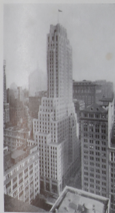
LEFCOURT NATIONAL BUILDING FIFTH AVENUE AT 43RD STREET Owner and Builder: A. E. Lefcourt Realty Holding Corp. Architect: Schreyer and Lamb
