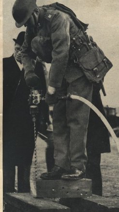
SPEED IS THE ESSENCE OF SERVICE in the Royal Engineers and when it comes to bridge building and other constructional work a high-speed drilling machine of this type proves an invaluable asset to the men.
