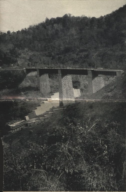
FOR LIGHT LORRIES ONLY: This bridge, lying just over fifty miles from the Chinese frontier, will have to be replaced if the Lashio route is to be available for heavy traffic
