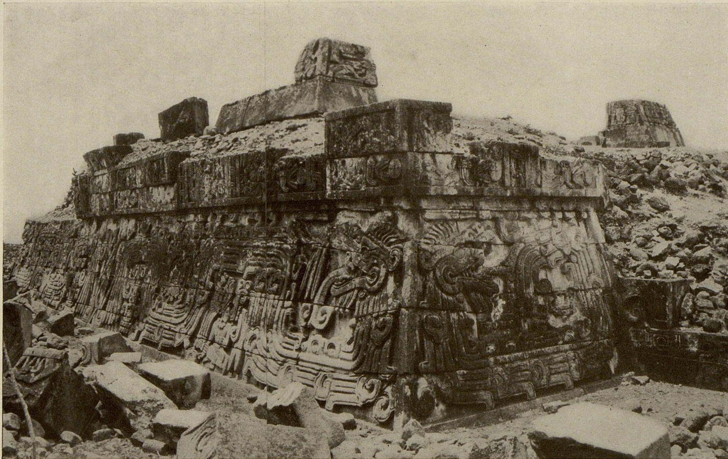
THE WALLS OF XOCHICALCO INCLINE FIFTEEN DEGREES FROM THE PERPENDICULAR, AND THE GREAT CARVED BLOCKS OF PORPHYRY WERE LAID TRUE WITHOUT CEMENT OR MORTAR.
